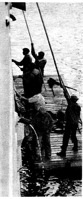
French workmen scrape the sides of the SPRINGFIELD as the water is pumped out of the Toulon drydock. The French workmen are doing most of the work on the hull.
